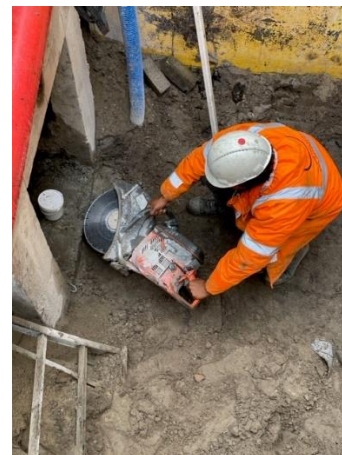
Figure 1: Power cutter and work posture
