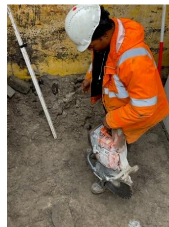
Figure 2: Employee trips as he gets up, whereby one of his hands shoots off the power cutter's handle causing the power cutter to drop down
